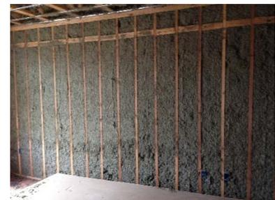
RockWool Filled Wall Cavity
